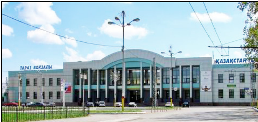
Figure 2.88: Taraz Railway Station.
