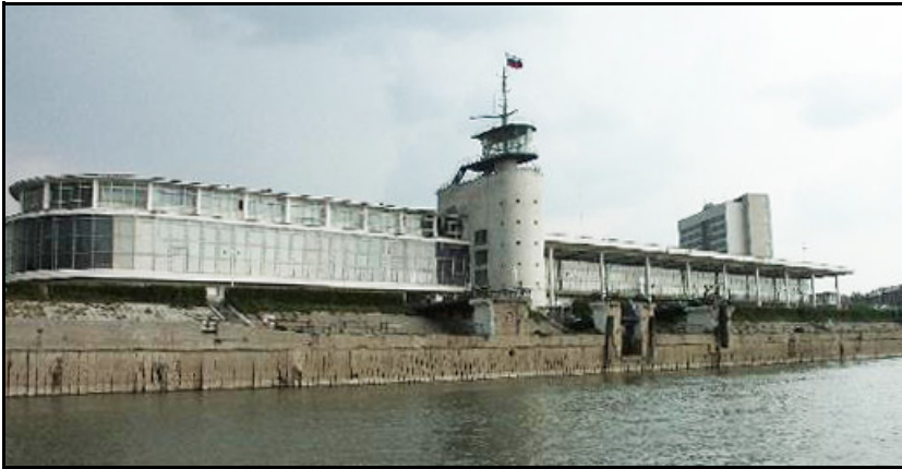
Figure 2.72: Hydroelectric power station on Irtysh River.
