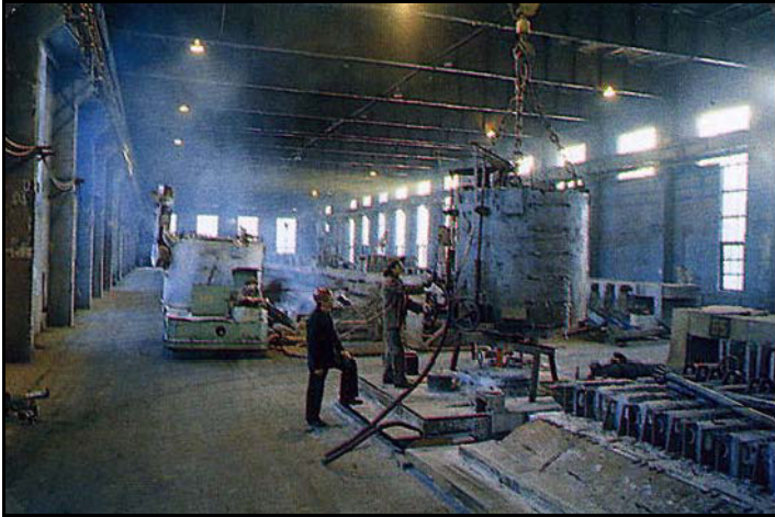
Figure 2.84: Magnesium electrolysis department.
