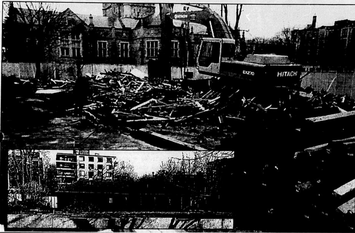
Ninety-five-year-old bowling club and green (below) sits empty (inset) with boards, called hoarding, put up last week. Above is crane flattening wood building in about 15 minutes Tuesday morning.
