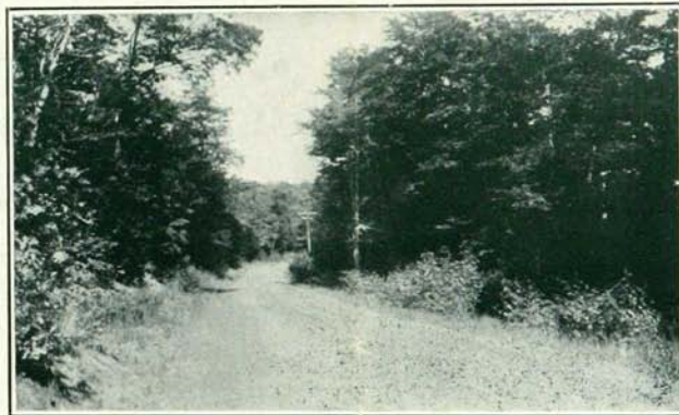
SCENIC VIEW OF ROAD AT STE. PETRONILLE
