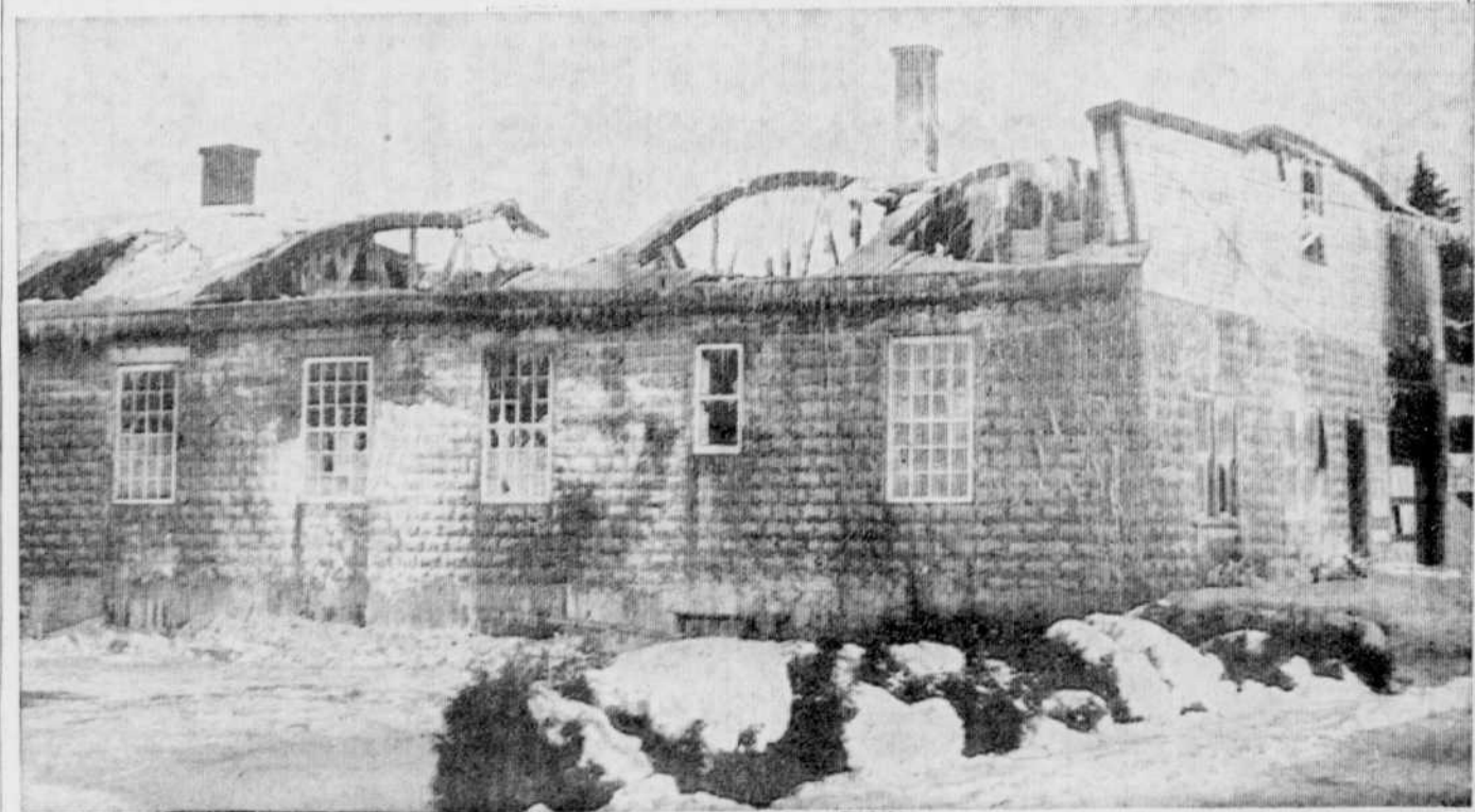
SCENE OF FIRE — A photograph taken early Thursday morning shows the burned-out shell of the B. Goyette and Son warehouse, 24 Bryant Street. One fireman was hospitalized and four others slightly hurt in the $125,000, three-alarm blaze. (Record Photo by Gerry Lemay)
