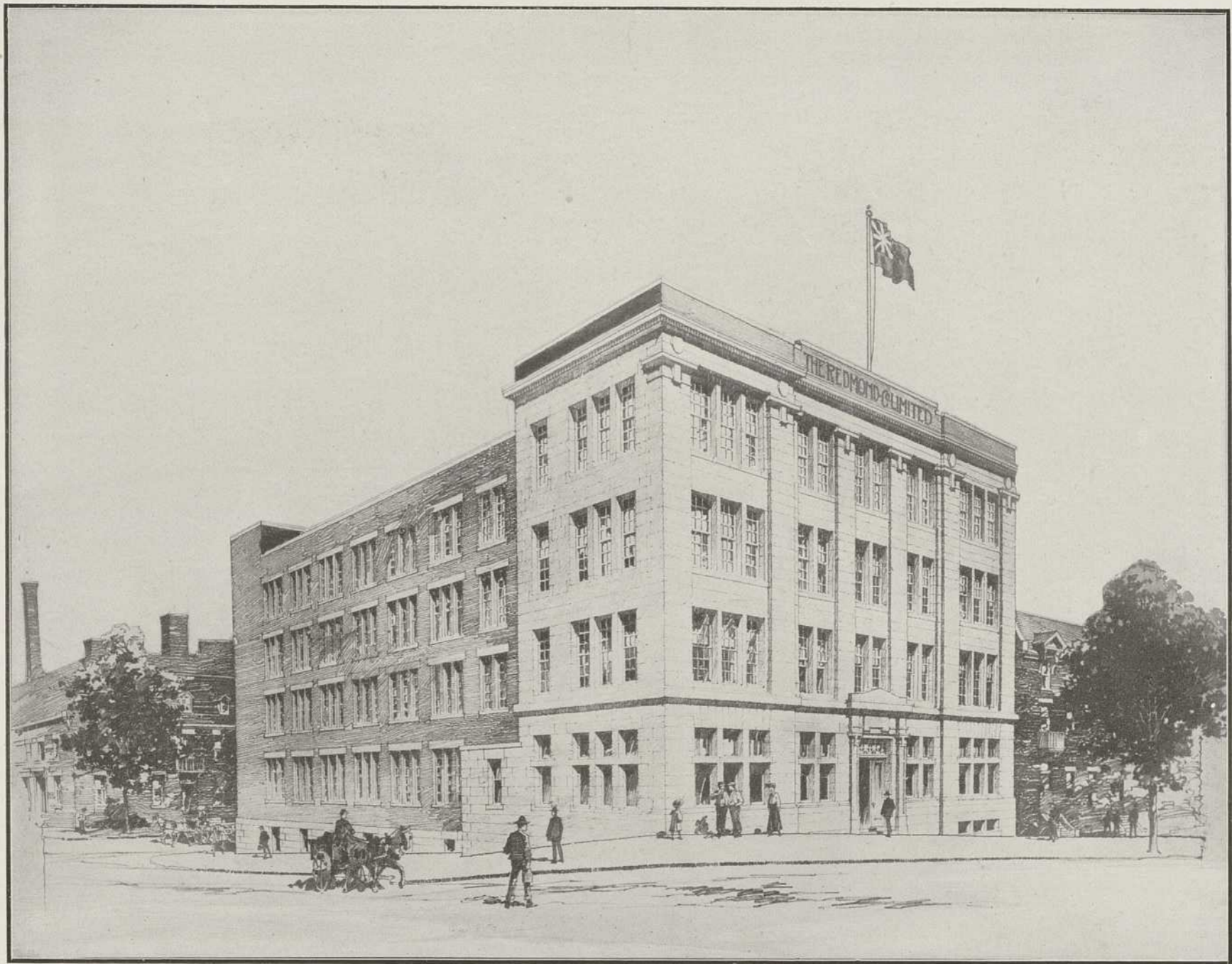
THE REDMOND BUILDING WHOLESALE HATS AND FURS
