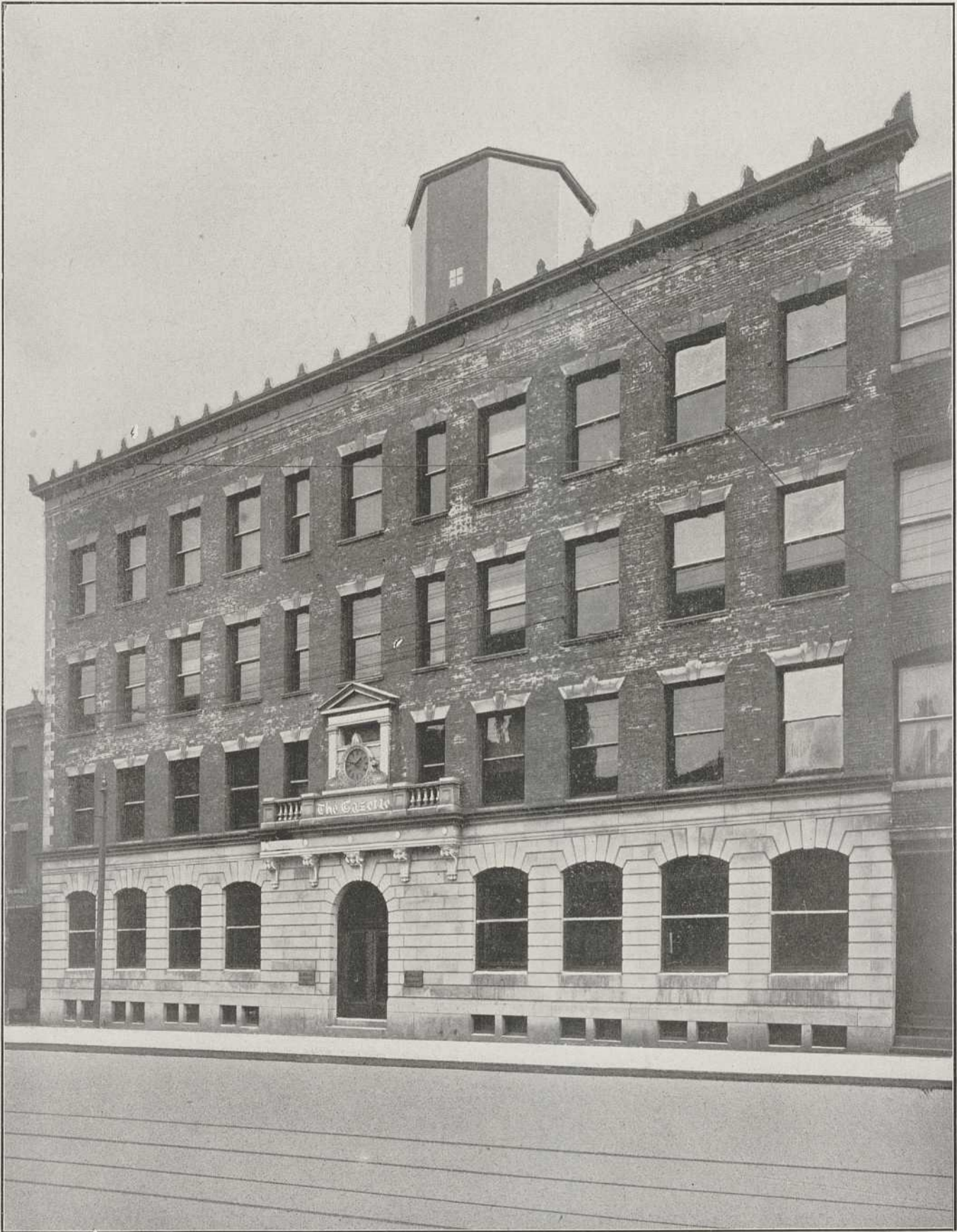
THE GAZETTE BUILDING
