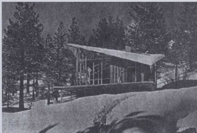
Figure 1. Cabine du ski
