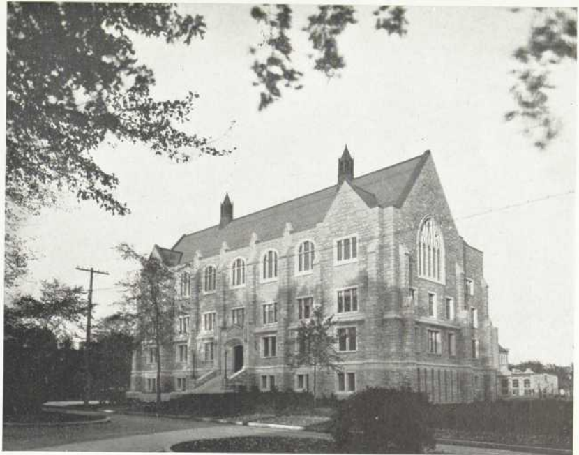
View from Southeast DOUGLAS LIBRARY, QUEENS UNIVERSITY, KINGSTON, ONT. Shepard & Calvin, Architects
