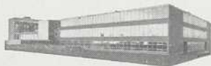
Collège Marymount, Sudbury, Ontario. Architectes: Fabbro et Townend. Entrepreneurs: Fassel Construction Company.
