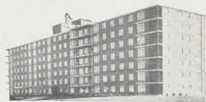
Park Tower Apartments, Winnipeg, Manitoba. Entrepreneurs: F. R. Lount Construction Co.
