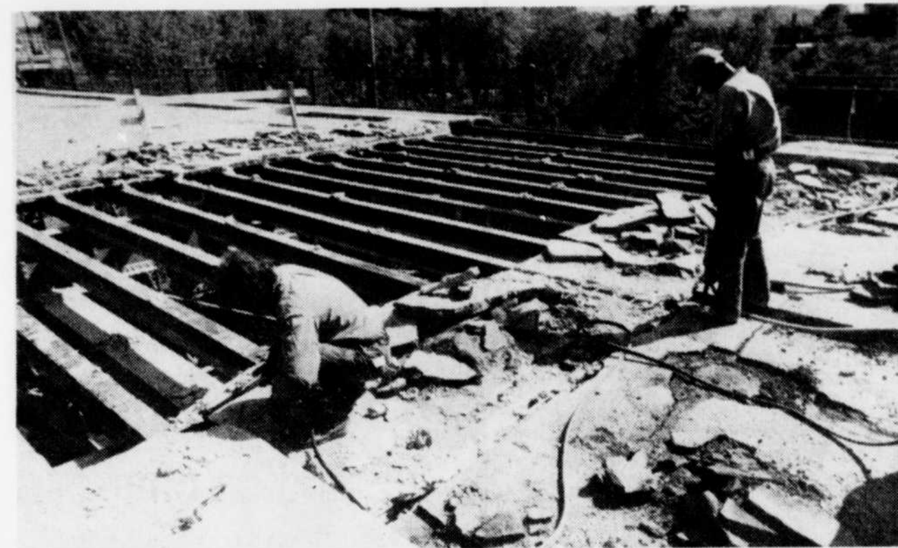
WOLFE BRIDGE — After being declared unsafe even for pedestrian traffic, Wolfe Bridge is finally being demolished by private contractors. Workers are seen here Tuesday as they cut the second section away from the bridge structure. The contractors must exercise extreme
