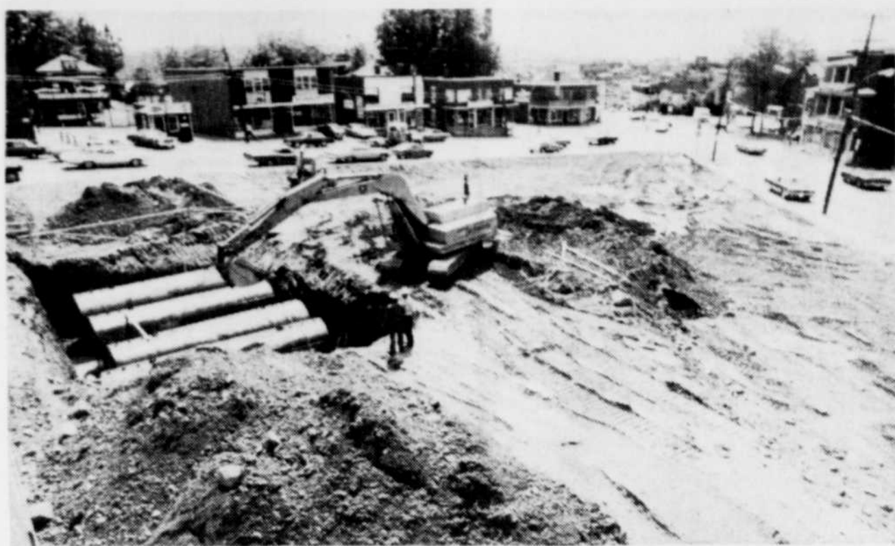
TANKS IN — The storage tanks for the proposed self service gas station to be built on the recently cleared corner of King and Papineau Streets were installed. The city intends to reorganise the King-Papineau-Murray intersection to ease traffic flow, which includes major
