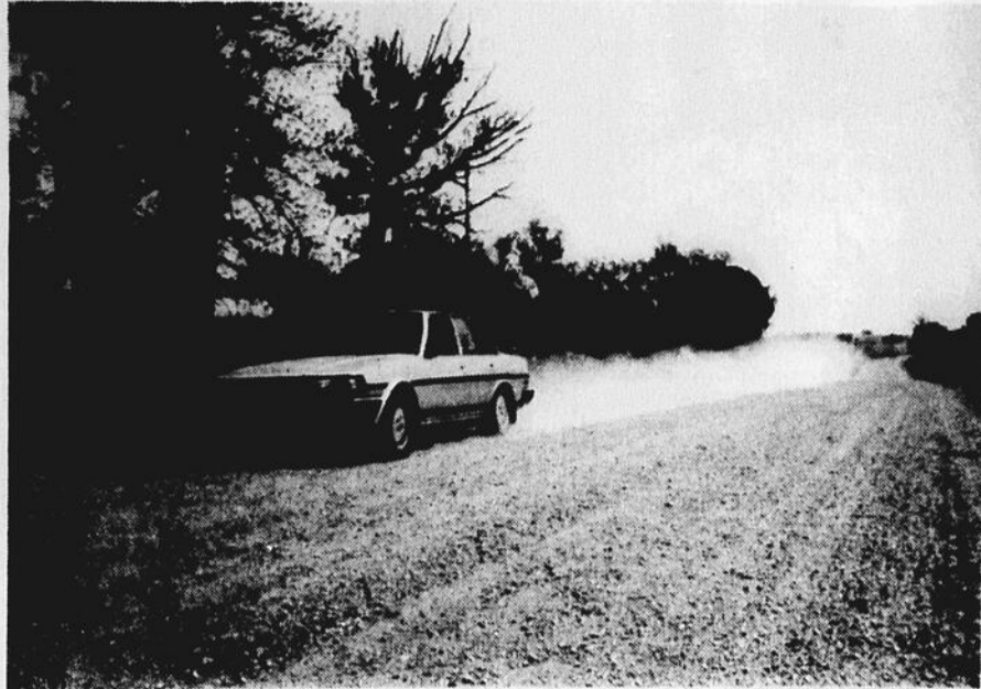
Since last summer, Route 202 has undergone widening and leveling just west of the Village yet the stretch of new road remains unpaved. During the dry spell recently, traffic created clouds of dust, annoying to those whose homes are adja-
