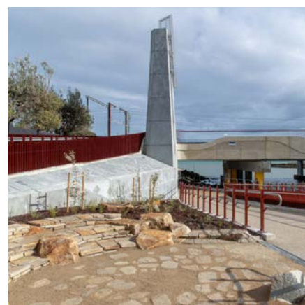
Photos courtesy Level Crossing Removal Project
