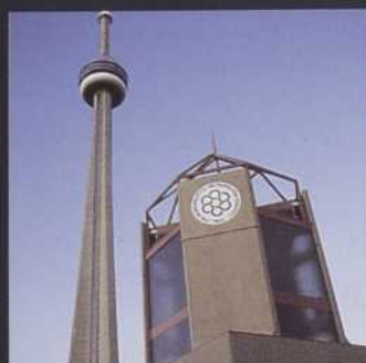
John Street pumping station
