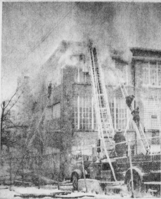
SCHOOL FIRE — Heavy smoke clouds pour out of the second storey paint shop window of the Sherbrooke Construction Workers' Apprenticeship Centre on Galt Street West, yesterday, where a noon hour fire originated. The 40-year-old building was heavily damaged by fire and water but the cause of the fire is not known as yet. Thirty firemen and eight fire trucks fought the blaze. Two Sherbrooke firemen were temporarily overcome by smoke.
