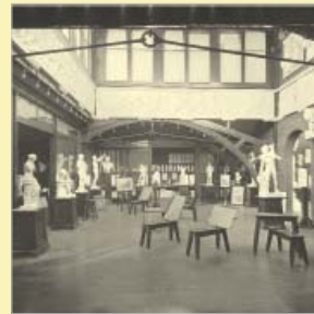
Architecture Department, Macdonald Engineering Building, circa 1900. Credit: W. Gourlie Blackie/McGill University Archives, PL0238652.
