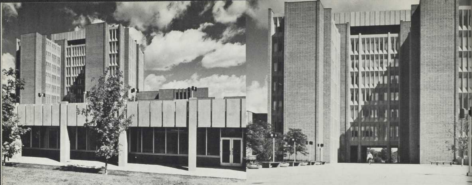
Architectes: Somerville, McMurrich and Oxley, Toronto Entrepreneur Général: Cooper Construction Company (Eastern) Ltd., Hamilton Entrepreneur Couvreur: Riddell Sheet Metal & Roofing Ltd., Hamilton
