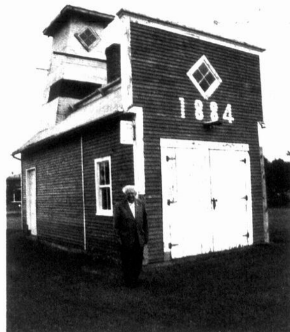
Gaetan Fortin stands before the original fire station from 1884 in Hemmingford. He has been working to restore the historical structure, which now sits next to the present day fire station just outside the Village (Photo: Sarah Rennie).
