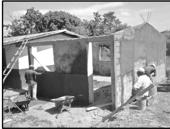
Storage room for new Las Pozas high school (Photo: Rodolfo Martínez)
