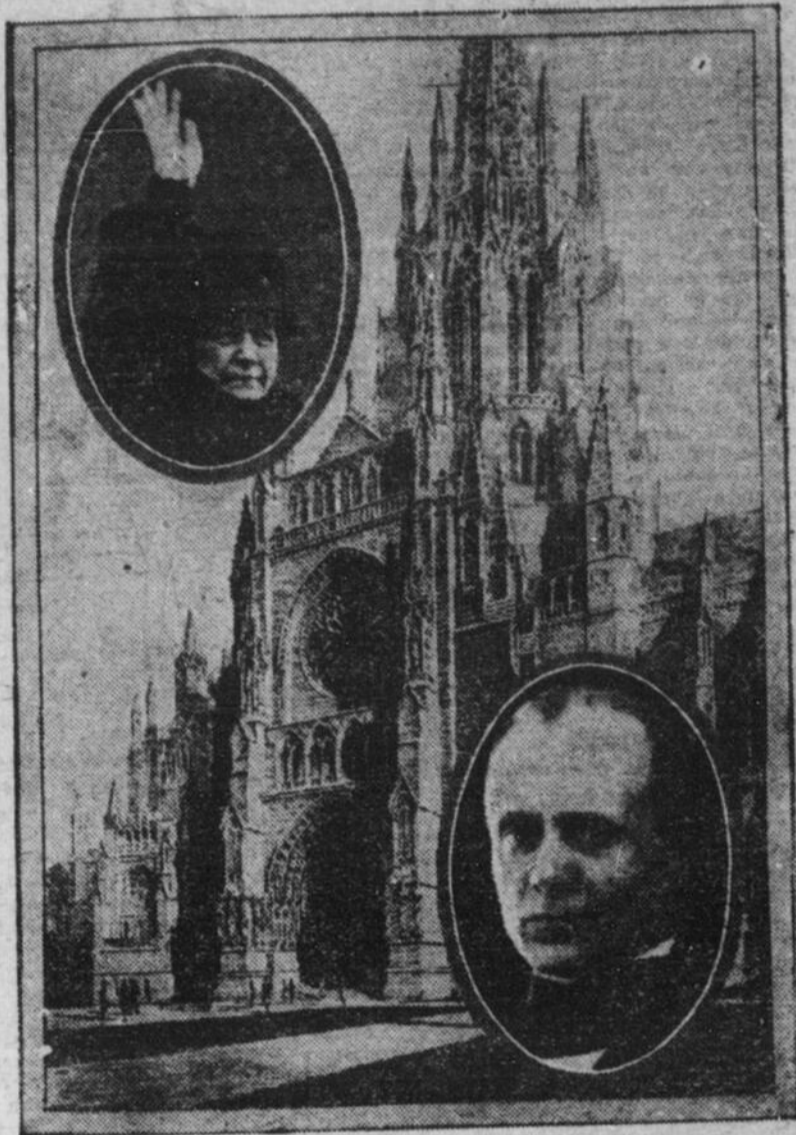
WOMEN UNDERTAKE BUILDING OF UNIT OF CATHEDRAL
