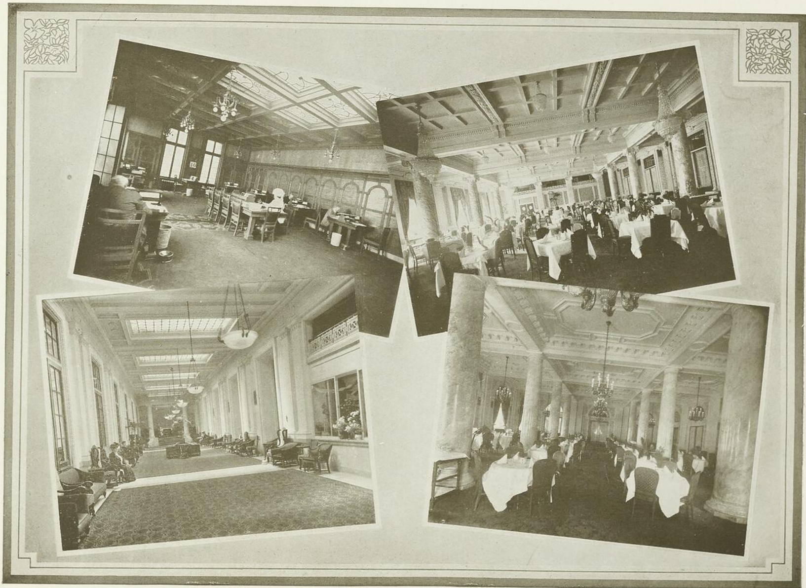
INTERIOR VIEWS, WINDSOR HOTEL
