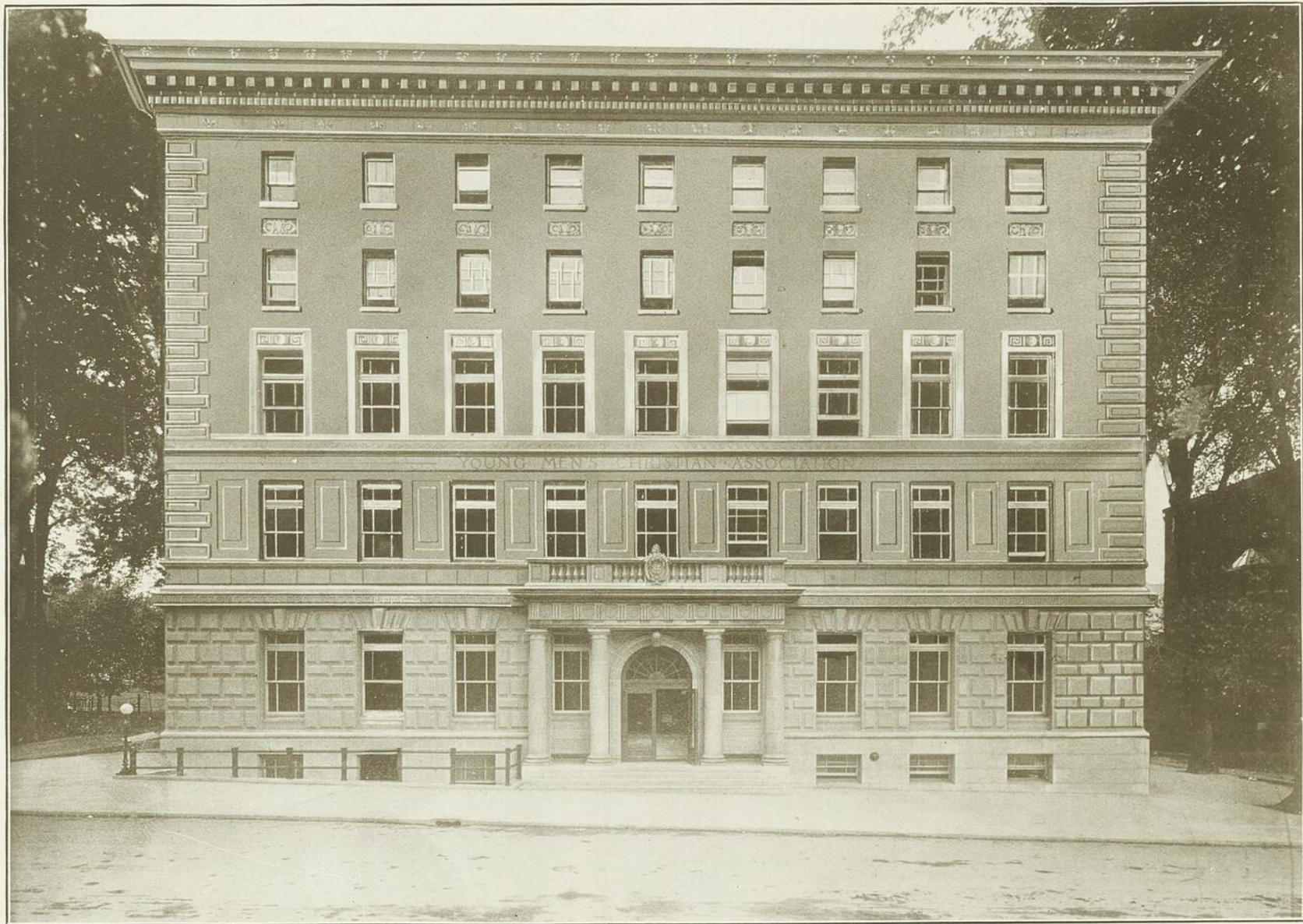
Y. M. C. A. BUILDING, DRUMMOND STREET
