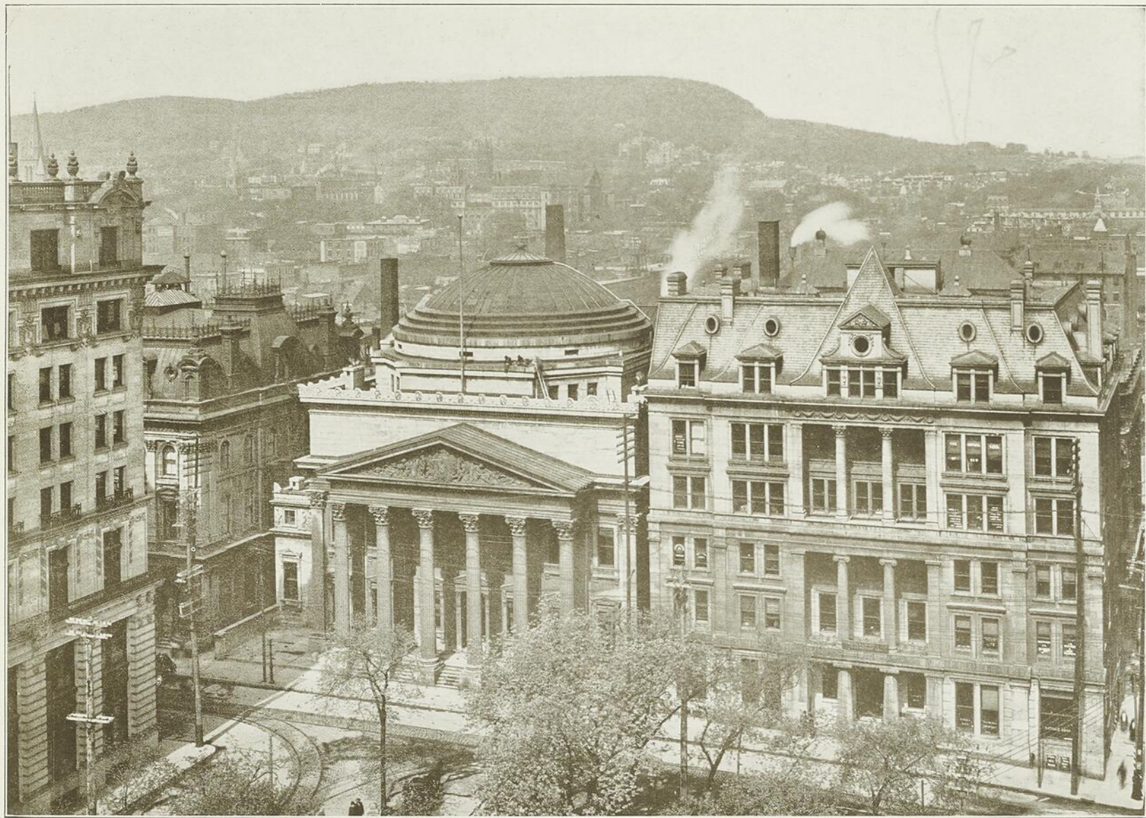
BANK OF MONTREAL AND ROYAL TRUST BUILDING
