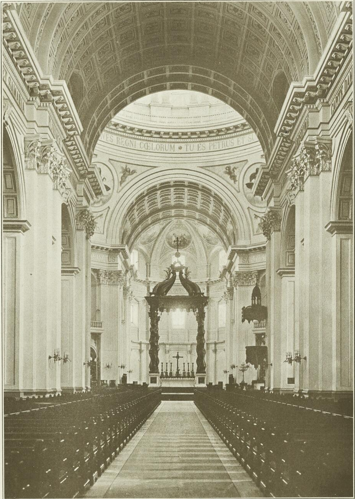
INTERIOR ST. JAMES CATHOLIC CATHEDRAL
