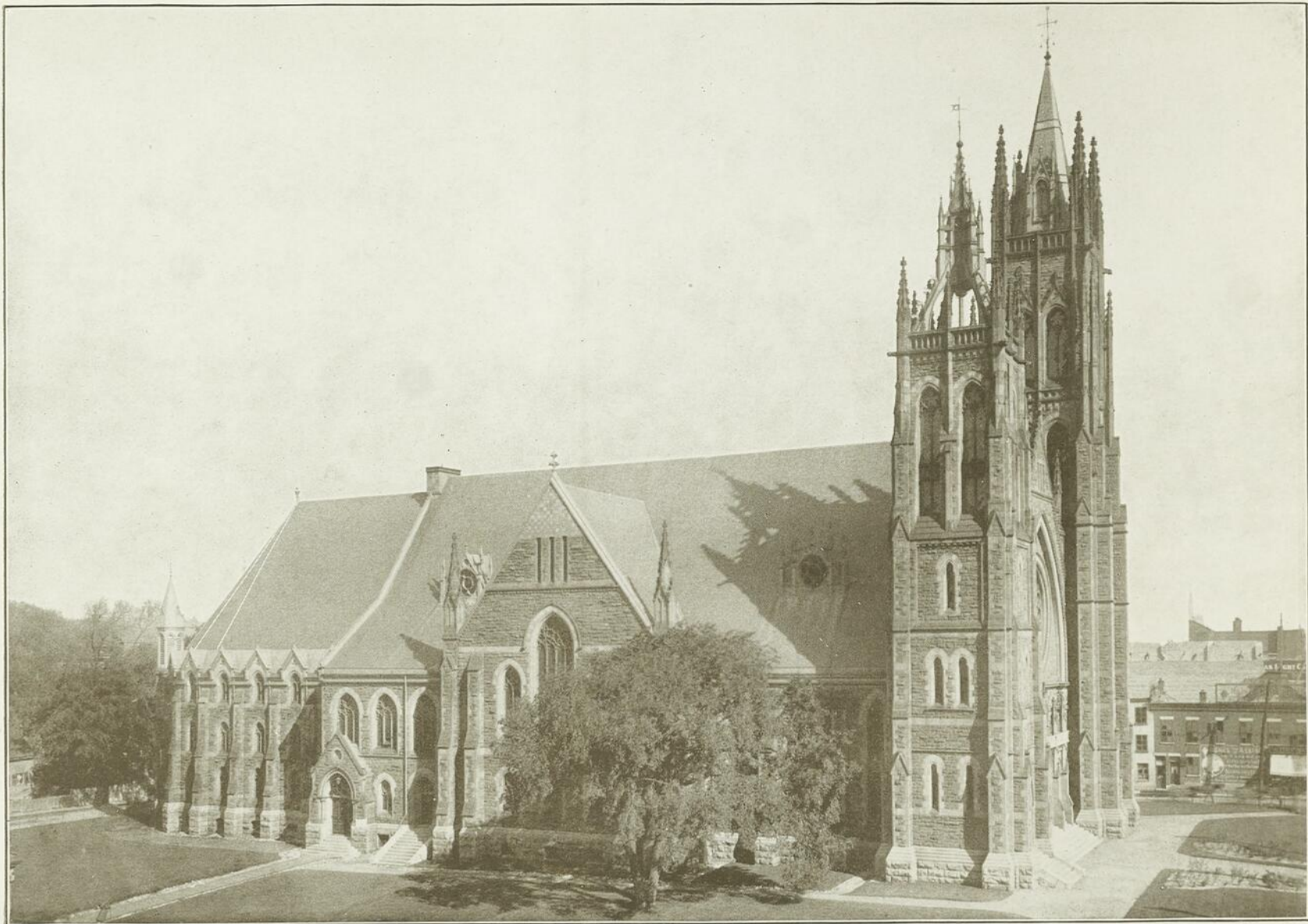
ST. JAMES METHODIST CHURCH, ST. CATHERINE STREET WEST
