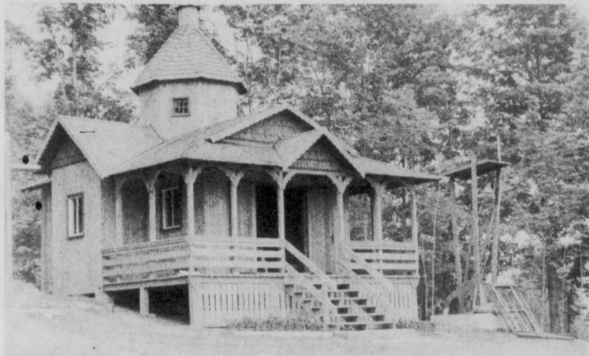
The Varokhta Ukrainian community's new chapel is made completely of wood. Members of the community paid for and built it themselves.
