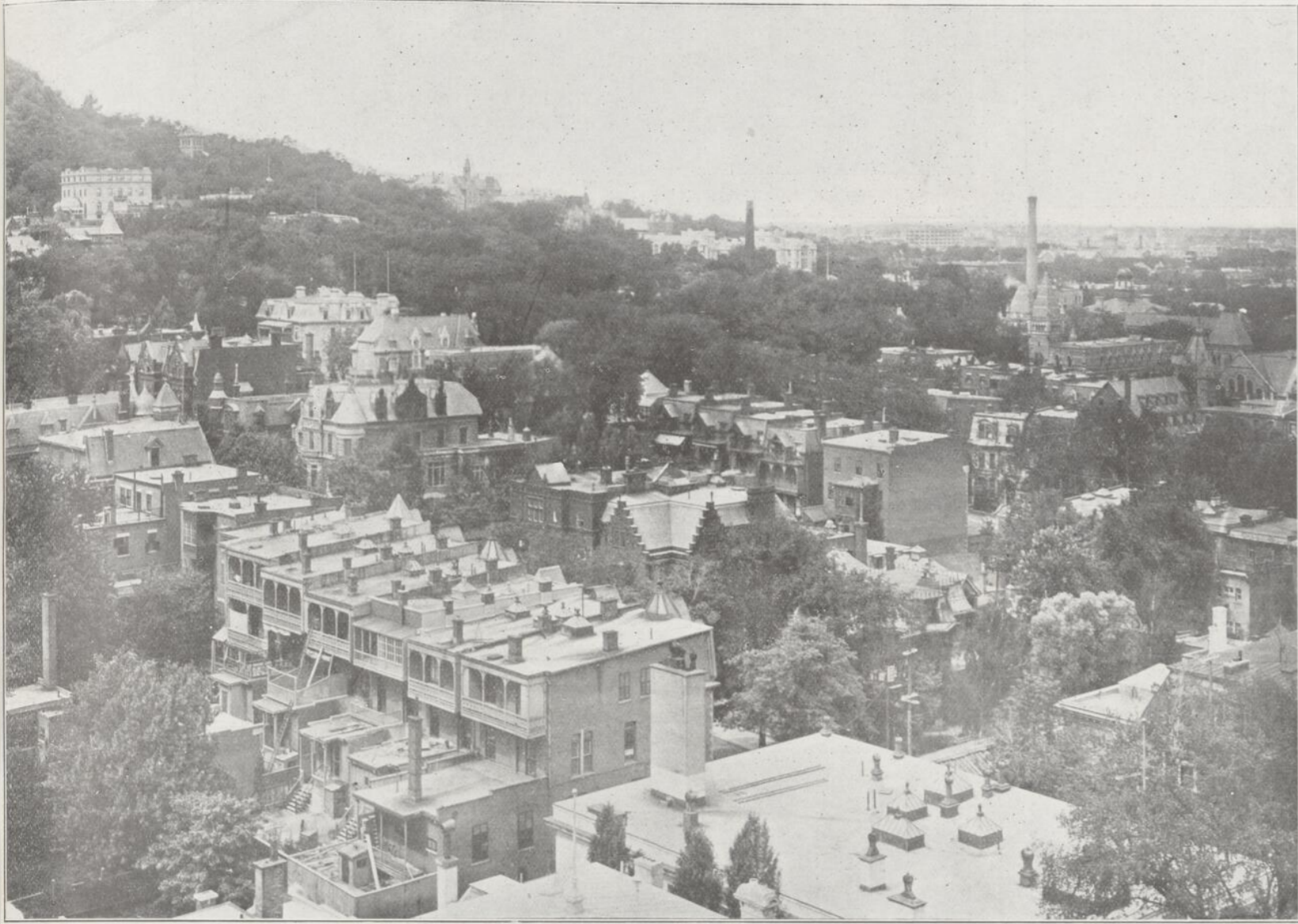
NEW VIEWS OF MONTREAL—Mount Royal and a portion of the residential section as seen from the roof of the new Ritz-Carlton Hotel. On the extreme left of the picture is the tower of "Ravensrag," the residence of Sir Montagu Allan. To the right, on the sky-line, are the Royal Victoria Hospital and the new Medical Building of McGill University. Further to the right is the dome of the Hotel Dieu, one of the oldest hospitals in Canada. In the foreground are some of the stately homes of prominent Montrealers, and in the centre (on the right) the Presbyterian College, and the Arts Building and the Peter Redpath Museum and Library of McGill University. (Photo by Kisseck.)
