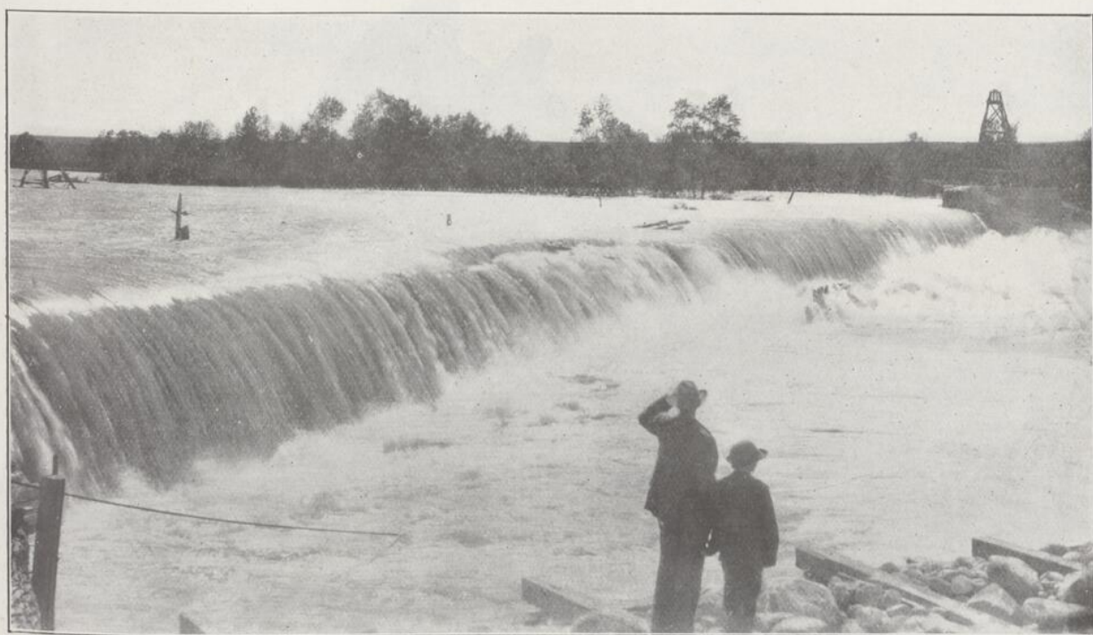
IRRIGATION IN THE PROVINCE OF ALBERTA—Dam across the Bow River. This ensures a constant head of water for one of the big irrigation ditches of Southern Alberta. (Photograph by Mrs. Edwin J. Baker, Glenview, Alberta.)
