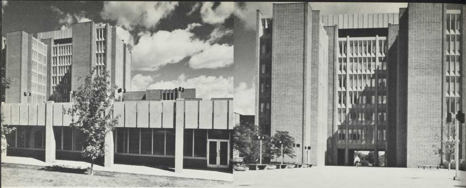
Architectes: Somerville, McMurrich and Oxley, Toronto Entrepreneur Général: Cooper Construction Company (Eastern) Ltd., Hamilton Entrepreneur Couvreur: Riddell Sheet Metal & Roofing Ltd., Hamilton
