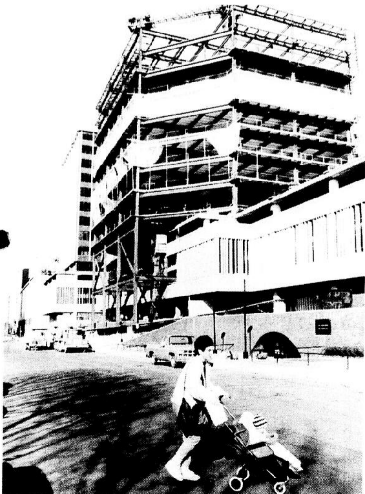
On the outside of the complex, the Alexis Nihon office tower has risen almost half of its proposed 18 storeys.
