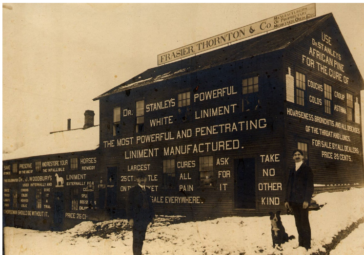
First Frasier, Thornton & Co. building in Cookshire, Que., circa 1903 Courtesy of Gloria [Frasier] Bellam
