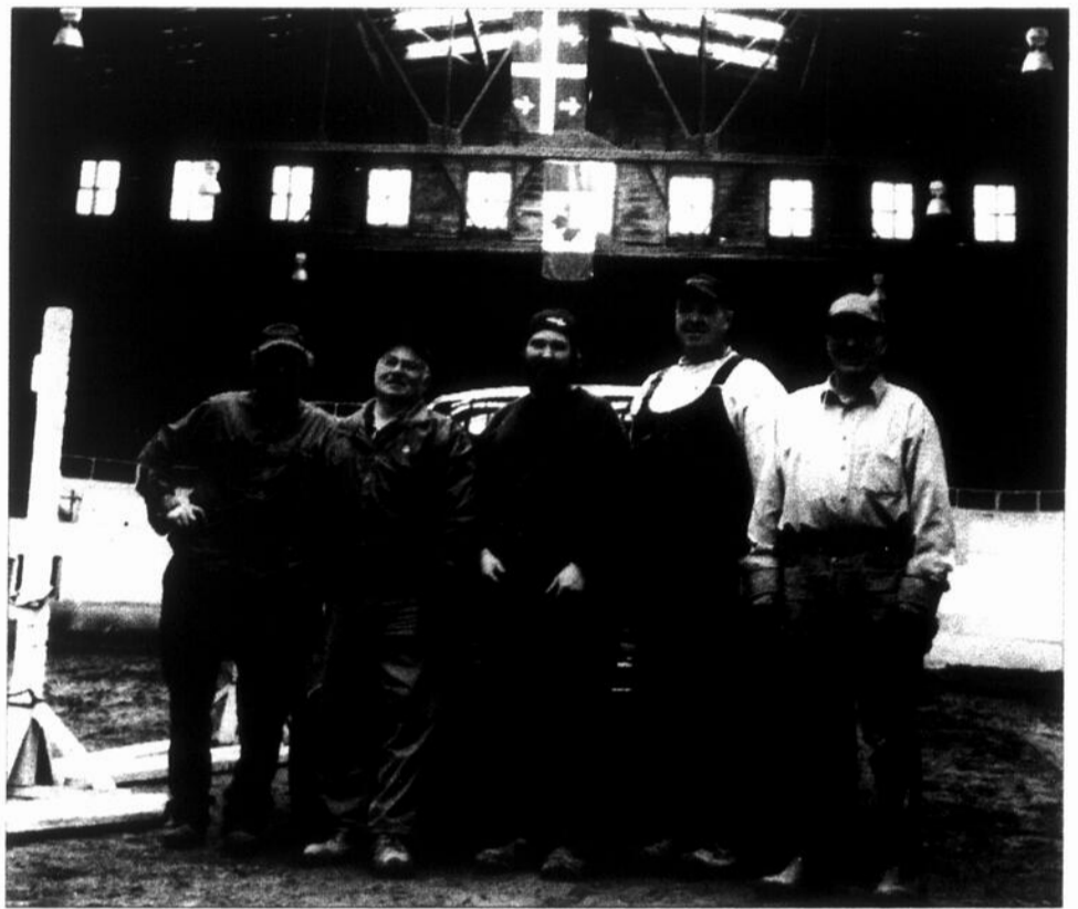
Volunteer and hired employees have been hard at work inside the Ormstown Arena repairing the gussets on the posts as well as steel reinforcement beams. The building now features a new upper roof that will keep the arena floor dry for years to come. Pictured here are Jack Lang, Carl Rember, Taylor Lang, Murray McClintock and Peter Finlayson. PHOTO: SARAH RENNIE
