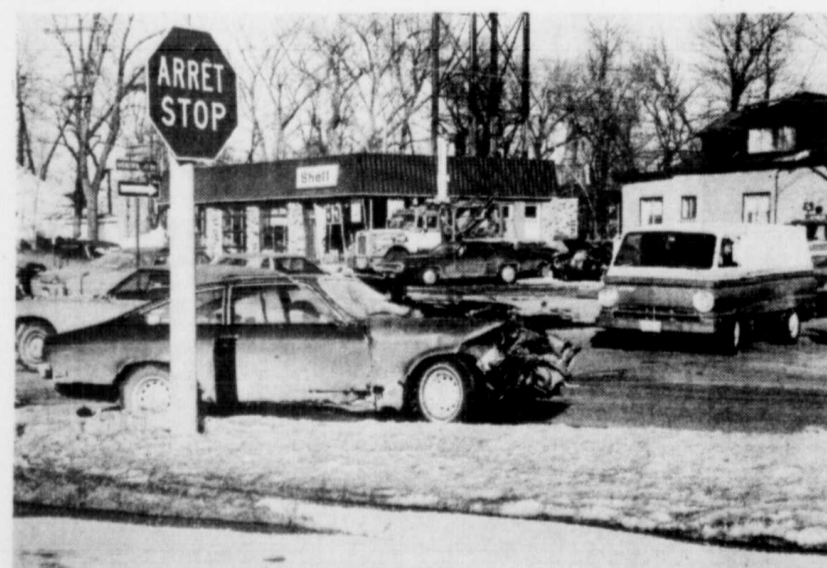
Never a dull moment when crossing Jacques-Cartier bridge. The car at the stop sign is in a state of shock. Corner Mercier & St-Laurent as we can see at the Shell station, it pays to have a big tow truck ready to be on the move fast and often. (Photo Bernard Brault)
