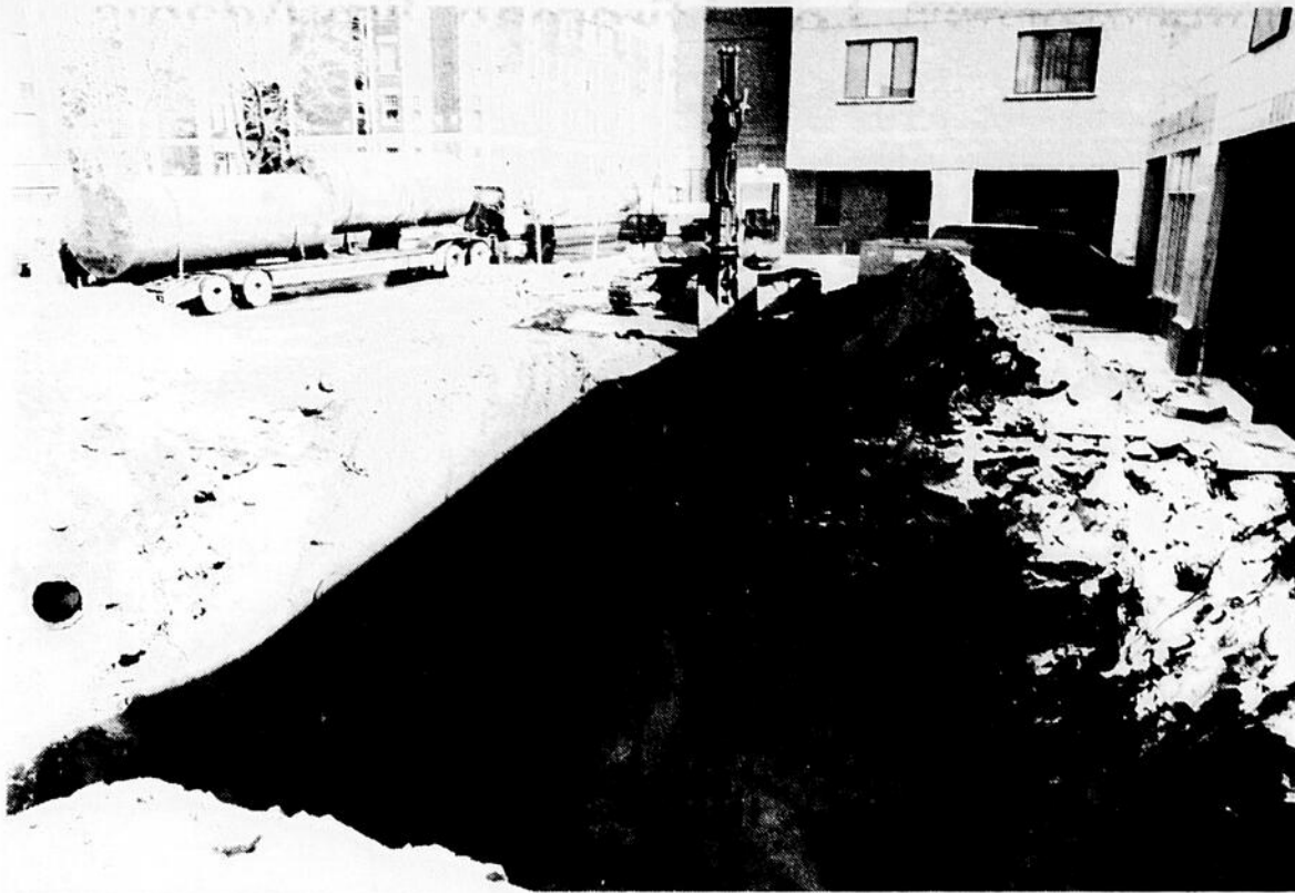
TANKS FOR THE MEMORIES: Men and machines dug up the old gasoline tanks (on truck in rear) of the former Timmins-Campbell garage on St Catherine street this week, the first stage of the demolition of the garage. Fairway Construction plans to construct a residence for seniors on the site.
