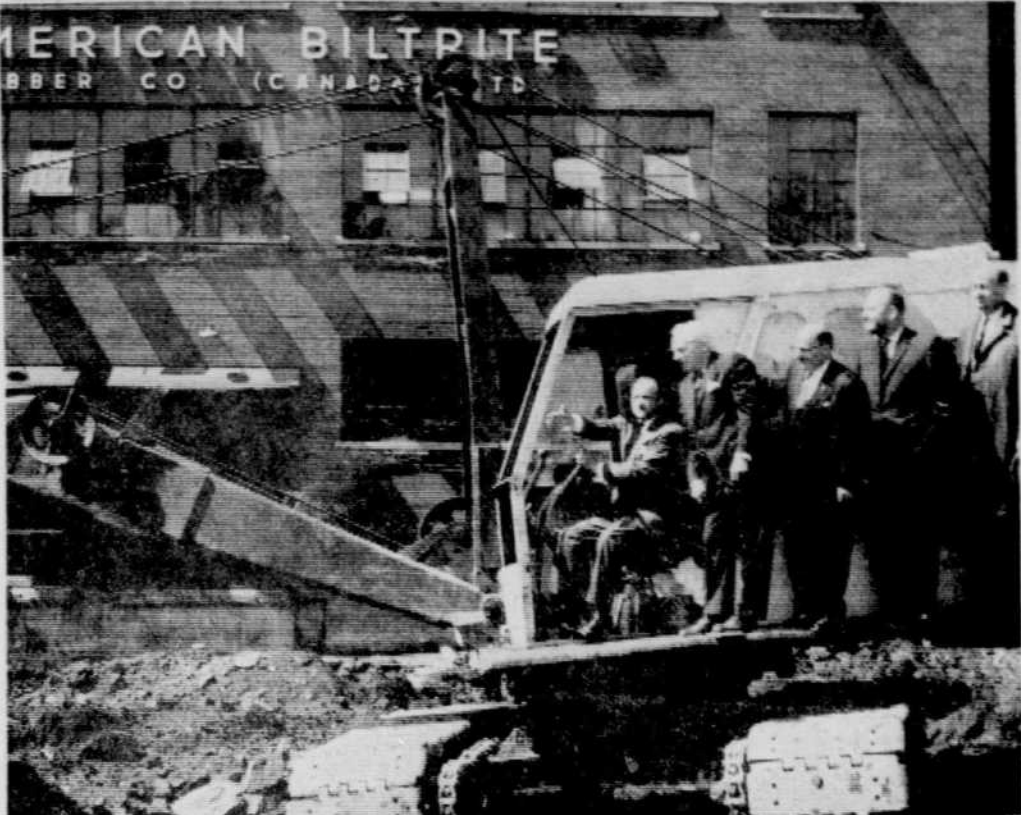
SOD TURNED —Mayor Armand Nadeau took over shovel controls from regular operator Red McIlarg Thursday morning to turn the sod for American Biltrite Rubber's extension to its plant overlooking the Magog River. Behind him at the ceremony is American Biltrite President C. Evans Joslin, and, from the left, architect Alphonse Belanger, Robert Belisle, secretary of the Sherbrooke industrial commis-
