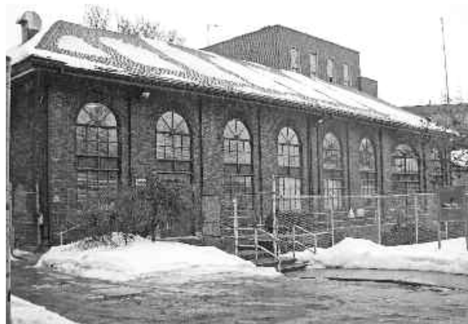
Hydro Westmount's principal building on Glen Rd.
