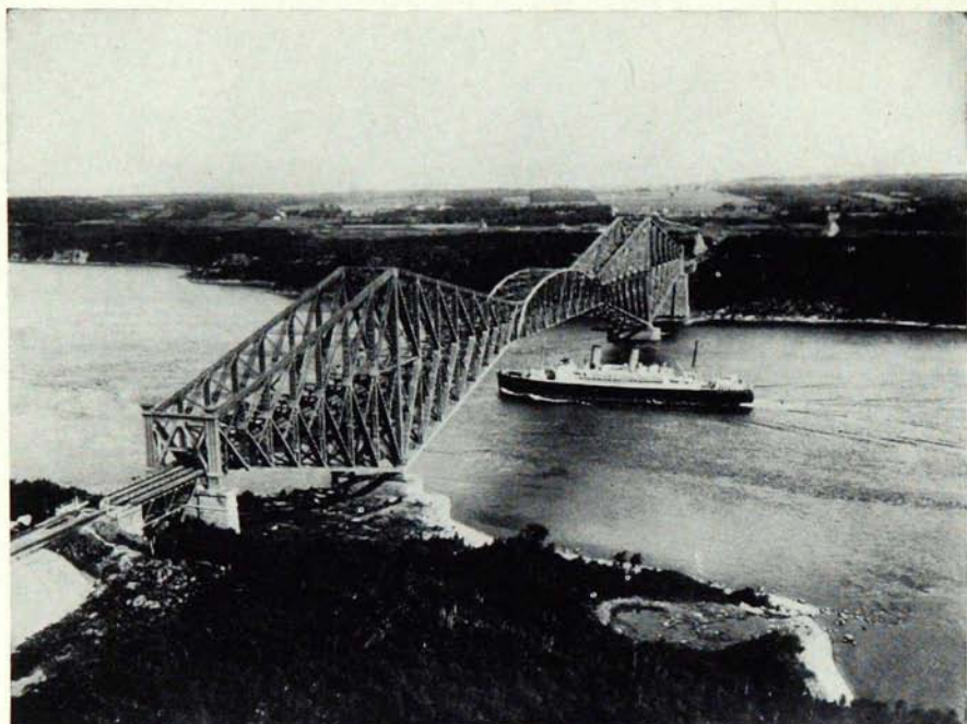
An air-view of the Québec Bridge, a famous feat of bridge engineering
