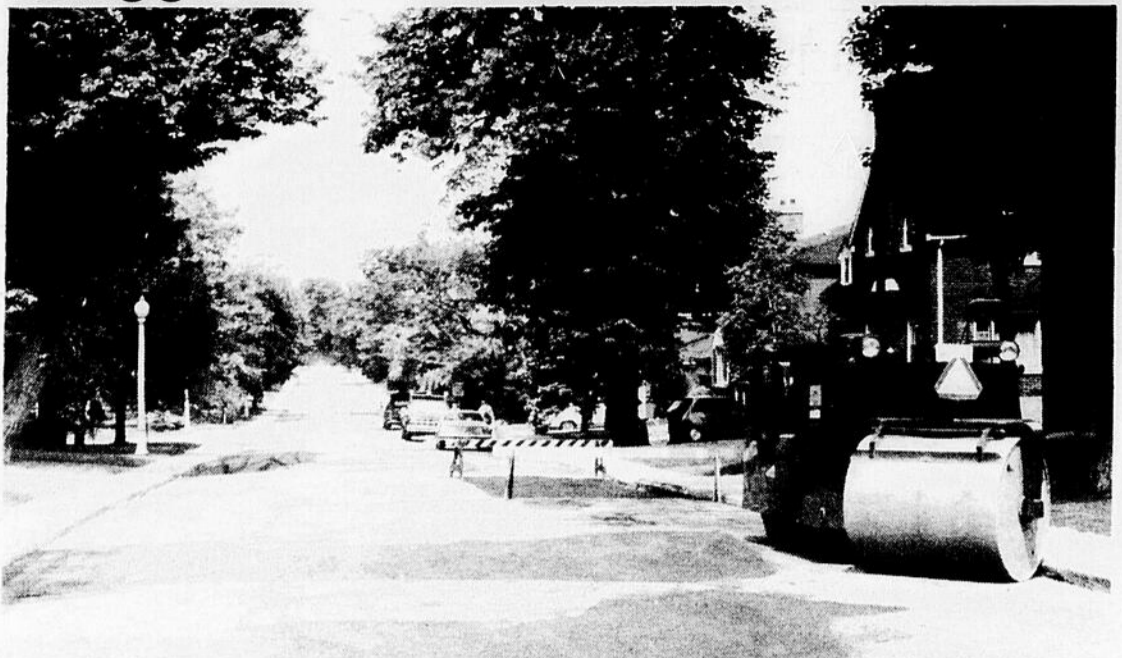
REPAIRING THE REPAIRS: Both sidewalk and road contractors had to be called back by the city to redo some of the work on Oakland avenue before resurfacing can take place.
