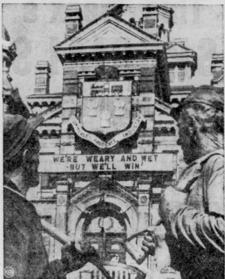
Pausing in their fight to stem the Red River flood menacing all of Winnipeg, two workers read the defiant message on the Winnipeg City Hall.
