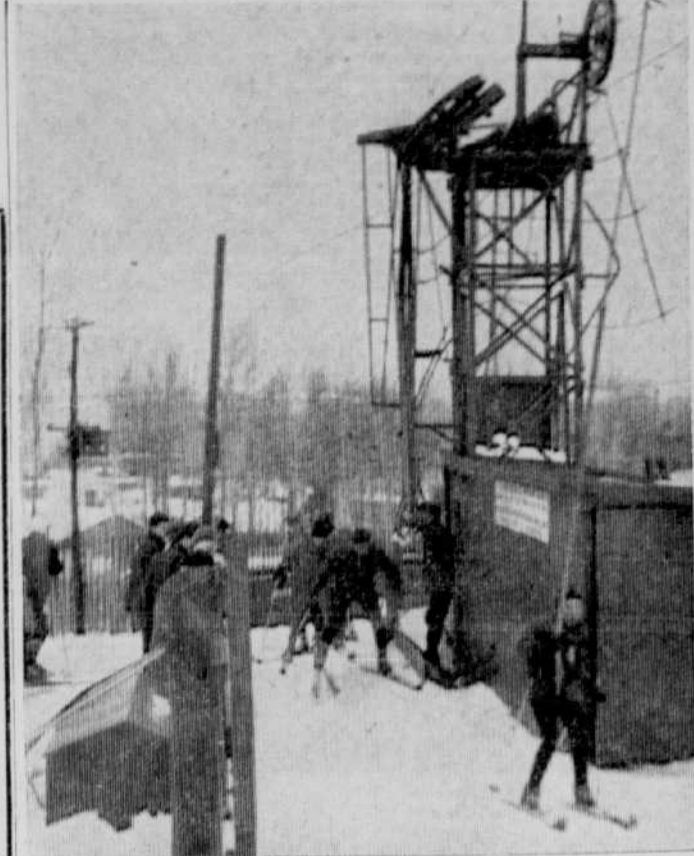
POMA LIFT — Sherbrooke's municipal ski centre has 1,800 foot long poma-lift with capacity of 1,000 skiers per hour.
