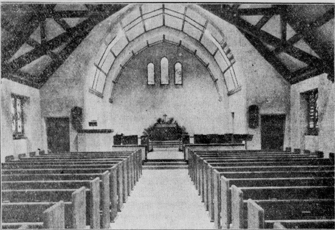
The top picture above shows the exterior of Saint Paul's Anglican Church, which is being consecrated this afternoon by His Lordship the Right Rev. Arthur Carlisle, Lord Bishop of Montreal. Below is an interior view of the new church. The altar pictured above is a temporary one to be replaced in a short time by a larger one.
