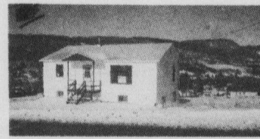
North Hatley: Sliding door from family room to patio, 4 bedroom bungalow, spacious living, panoramic view.
