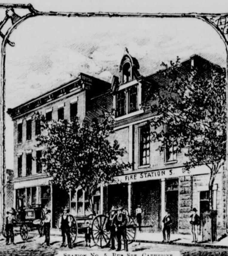
STATION No. 5, RUE STE. CATHERINE
