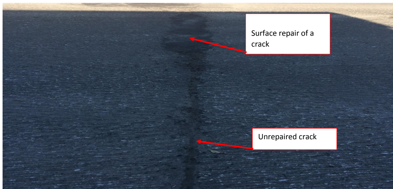
– Photo 2 taken by the OIG on September 17, 2015, on Monselet Street, illustrating an unrepaired defect.
