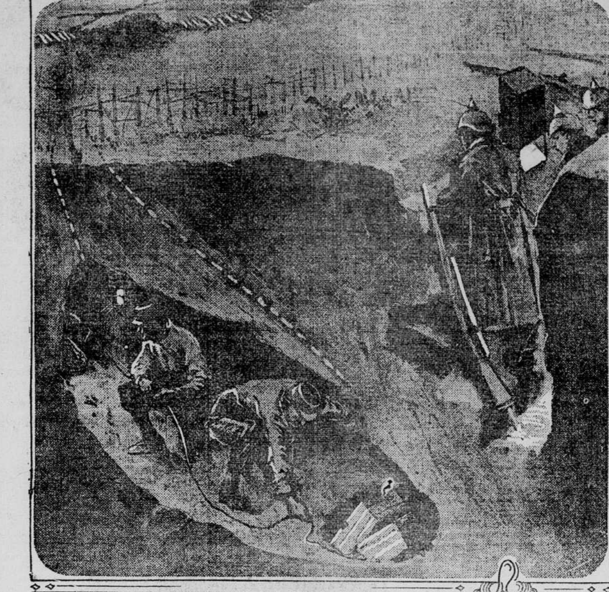
Taking a trench by assault is extremely dangerous, and costly under modern conditions of warfare and the greatest danger is from under the earth. The sketch shows a party of French sappers who have burrowed through the earth between the two lines of trenches and are connecting an electric wire with the dynamite which they have placed under the enemy. When the dynamite is exploded the trench will be rushed by the French infantry. Both sides engage in sapping operations and the first to reach the opposing trenches through their underground galleries will be victorious.
