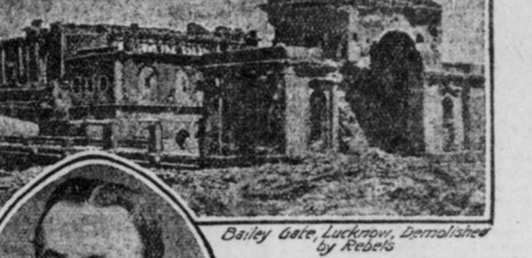
Bailey Gate, Lucknow, Demolished by Rebels
