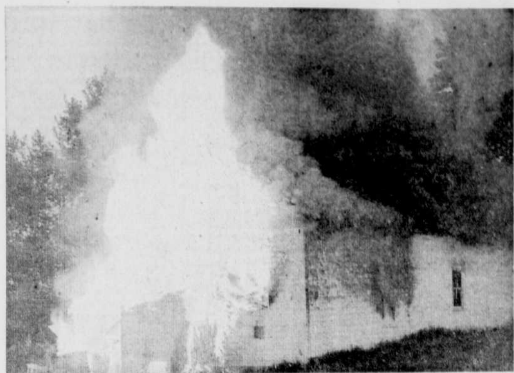
FIERY RUIN — Smoke and flames can be seen pouring out of the Rene Guenette house and neighboring shed at 302 Williams Street, Thursday evening. The $6,500 fire, believed to have been caused by an exploding oil drum, destroyed the two-story shed and gutted the house. Mrs. Guenette and her three children were in the house at the time of the fire, but they escaped and no one was injured. (Record Photo by Studio Eclair)
