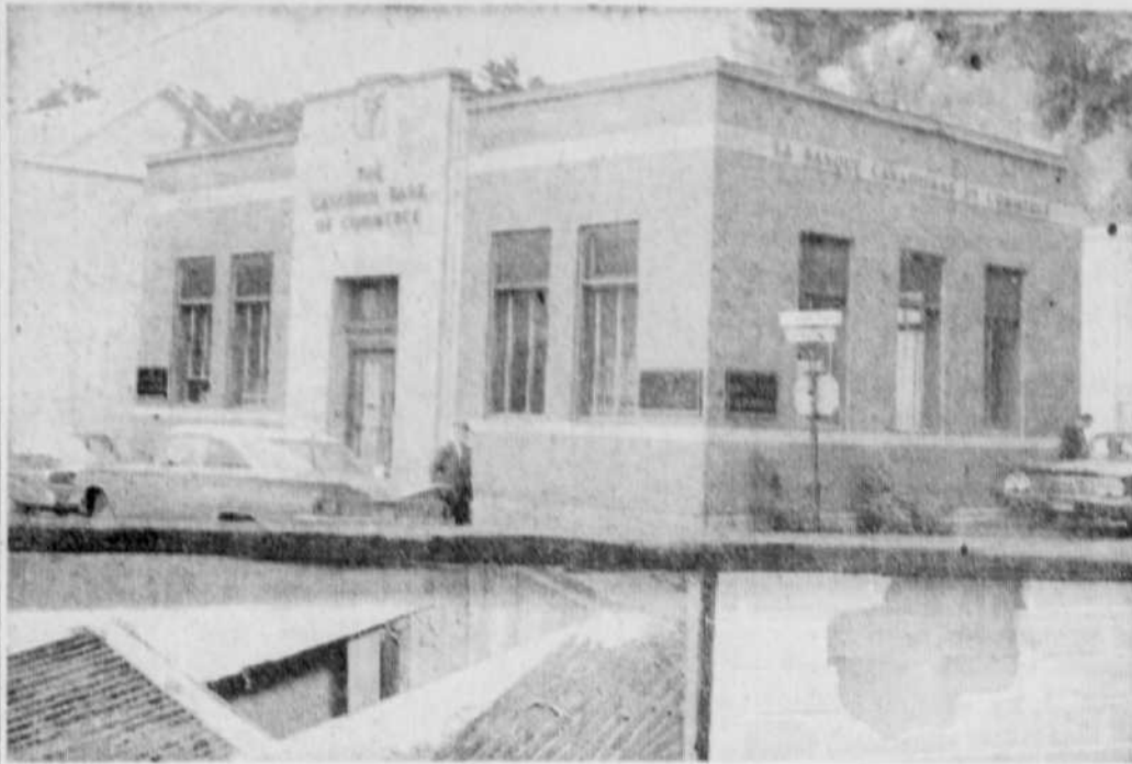
ATTEMPTED ROBBERY — Above is the Bedford Branch of the Canadian Bank of Commerce, located at the Main-Pine Streets corner, where thieves, early Saturday morning tried to gain entrance to the vault. Lower left is the basement window through which the thugs gained entrance to the basement of the establishment. Lower right is the hole they made with a sledge hammer at the rear of the building. (Record Photo by Studio Eclair)
