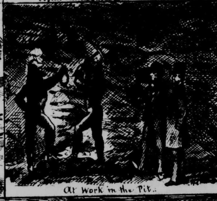
At Work in the Pit.
