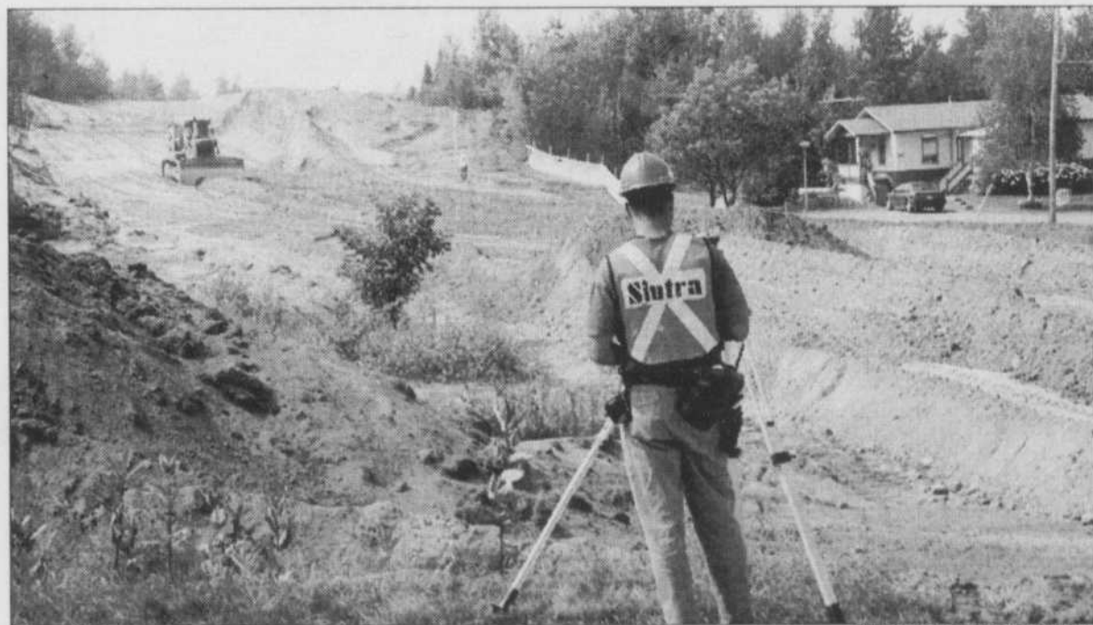
Surveyor and bulldozer shape the roadbed west of Craig Road.
