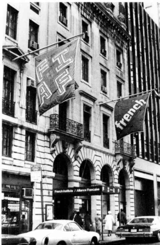
THE FI / AF BUILDING, 22 East 60th Street, New York, NY
