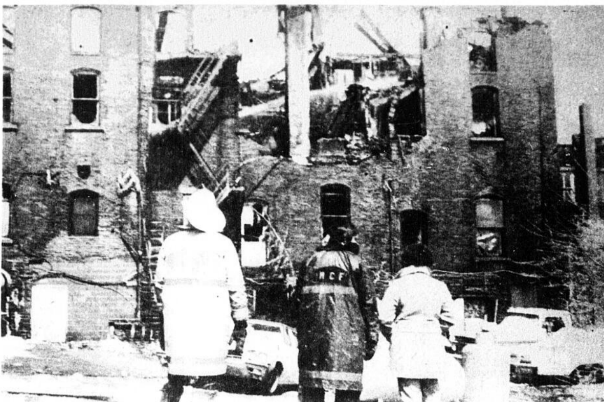
Malone firemen survey wreckage of Easter Saturday fire.
