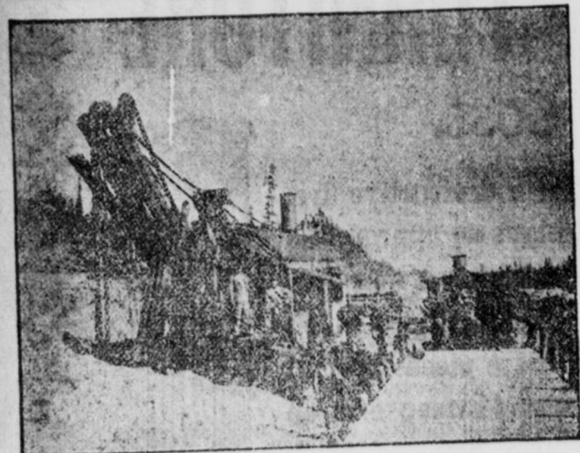
SHOWING STEAM SHOVEL LOCOMOTIVE AND FLAT CAR.
