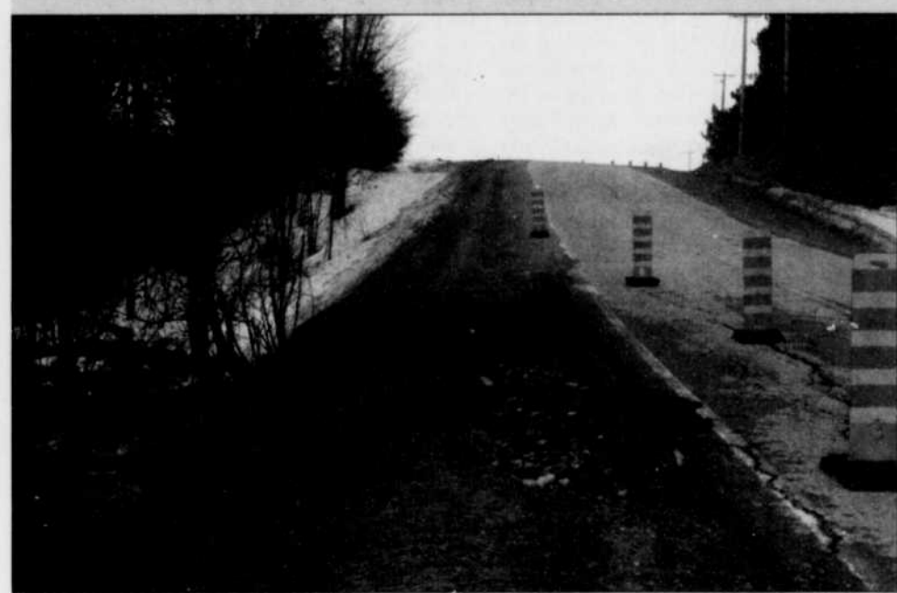
A culvert on the Bristol Road in Bristol nearly overflowed causing a wash-out concern for the Quebec Ministry of Transport on last week Wednesday.
