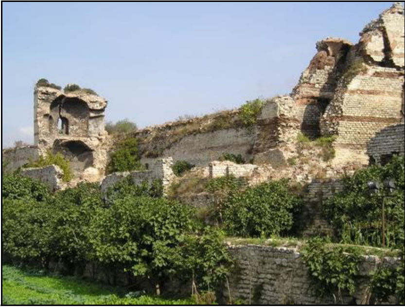
Figure 2.58: Part of the original wall.
