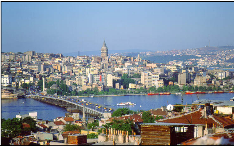
Figure 2.26: Bridge connecting İstanbul and the Golden Horn.
