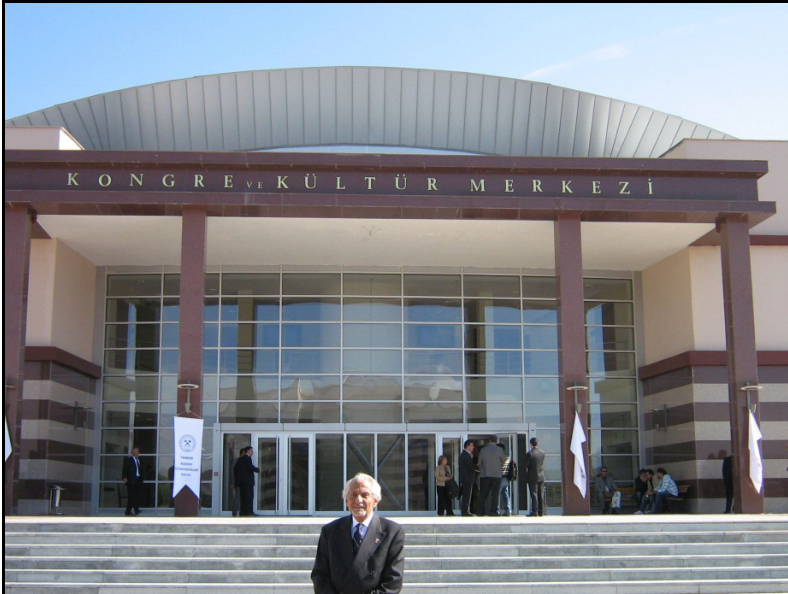
Figure 2.129: Convention Centre at Osmangazi University.
