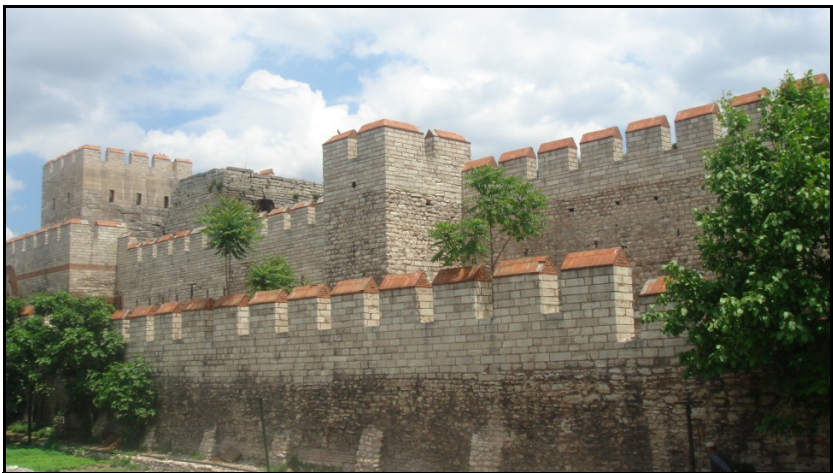
Figure 2.59: Part of the restored wall.
