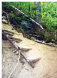
The old deteriorated trail.
