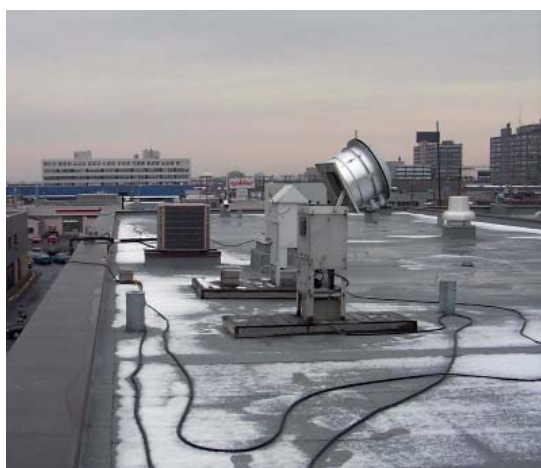
Monitoring station 44 (Saint-Michel)
