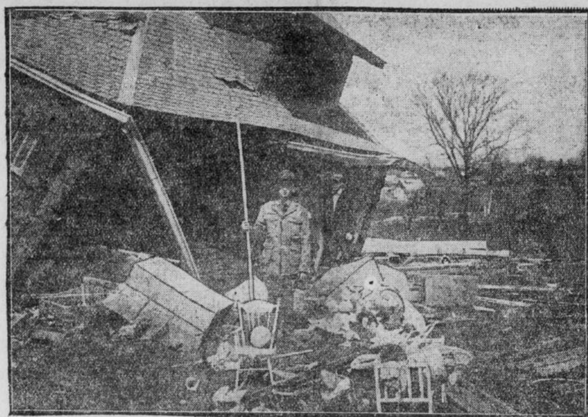
Twelve buildings were completely destroyed and a number of persons injured in a tornado which recently swept the little town of Silver Springs, Md.
